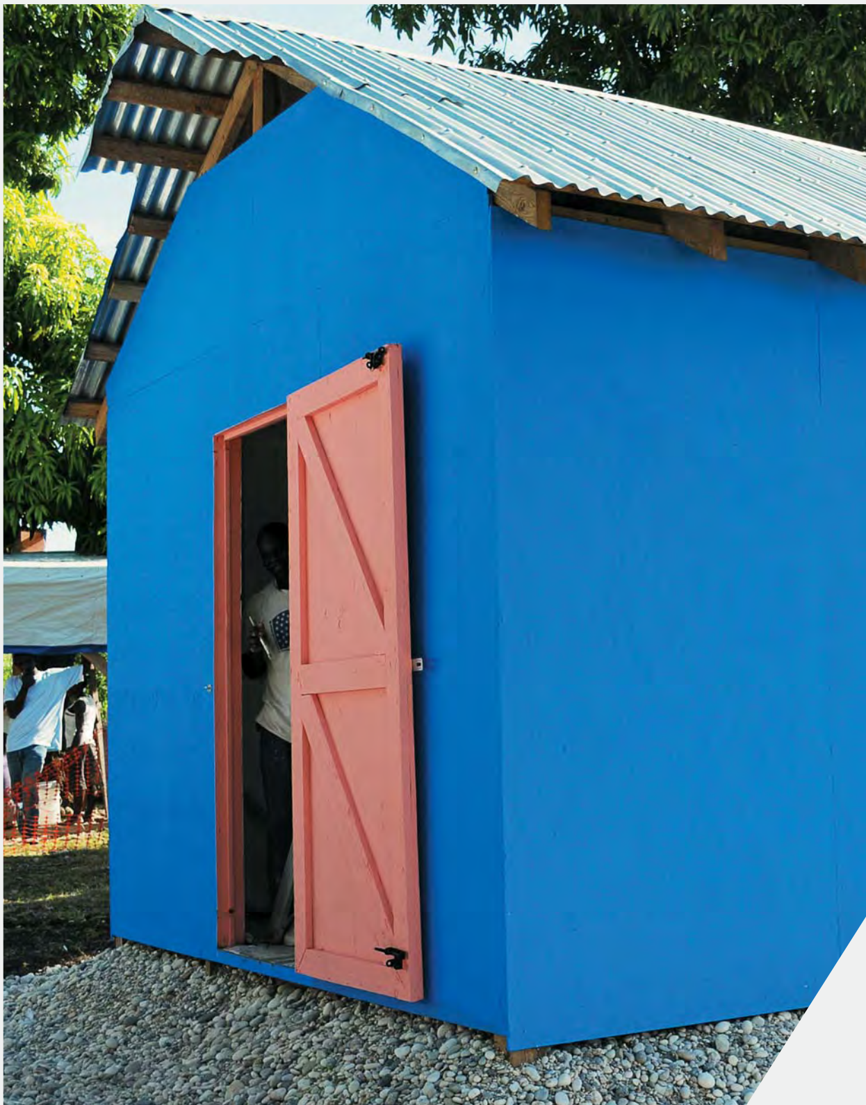
A COMPLETED CANADIAN RED CROSS SHELTER.
